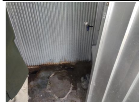
Figure 3 – Toilet covered with concrete to stop usage due to incorrect construction in Petobo Shelter
