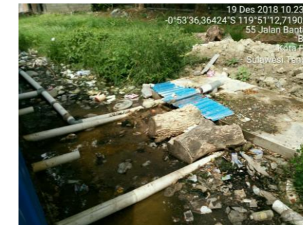
Figure 7 – Puddled water due to disconnected blackwater pipe in Masjid Agung Shelter
