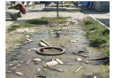
Figure 8 – Puddled water due to septic tank overflow in Bangsa Shelter
