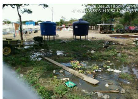
Figure 6 – Puddled water due to bad placement of water tank in Layana Shelter
