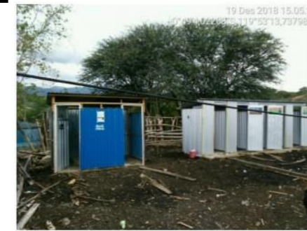
Figure 4 – Toilets built on unstable soil in Layana Shelter
