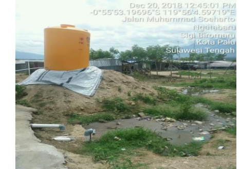
Figure 5 – Puddled water due to septic tank overflow in Petobo Shelter
